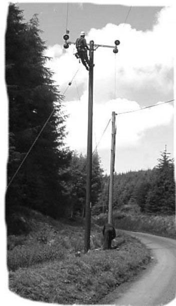
Prosiect Trydan, Cwm Brefi Electrification Project, Cwm Brefi
